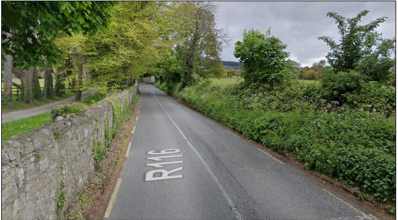
Figure 12-11 Ballybetagh Road R116 Typical Road Section (source: google maps)
